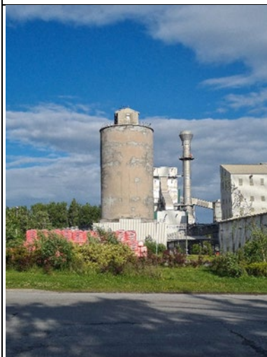
Plate 21: Example of industrial buildings within the active part of the wider site
